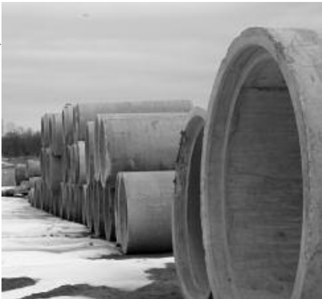
Rows of sewer pipes behind Eastwood Towne Center await burial.
